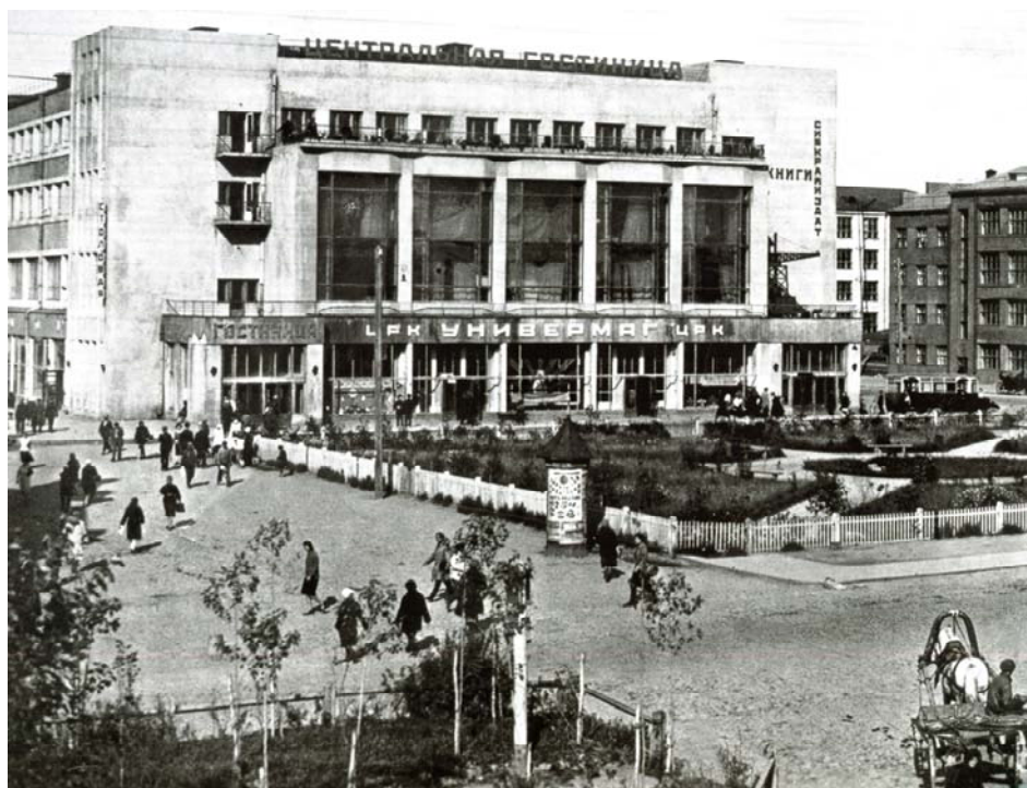
Доходный Дом Commercial Apartment Building
